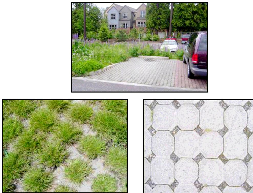
**Figure 41: Examples of Permeable Pavers**
