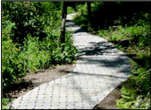
**Figure 16: Sidewalk with a Permeable Paver Surface**
