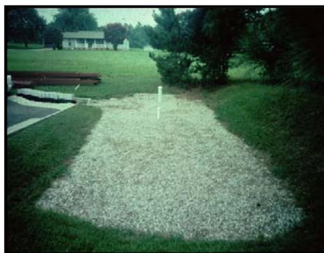
**Figure 39: Infiltration Trench**
