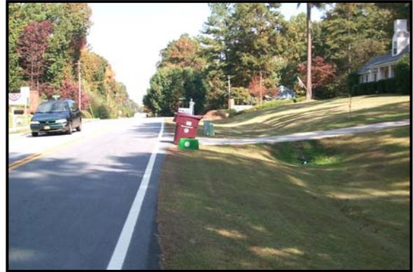
**Figure 33: Examples of Open Vegetated Channels**
