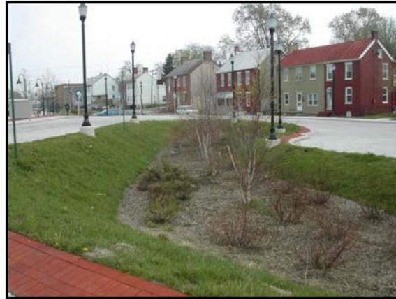
**Figure 36: Example of a Bioretention Facility Along Roadway**
