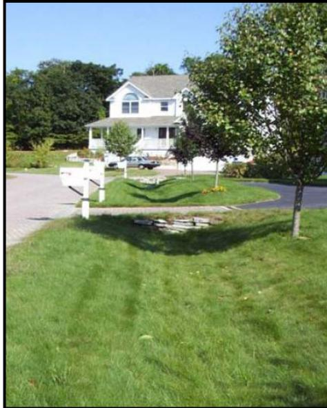
**Figure 34: Another Example of an Open Vegetated Channel**
