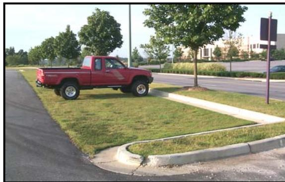
**Figure 28: Grass Paver Used for Parking**
