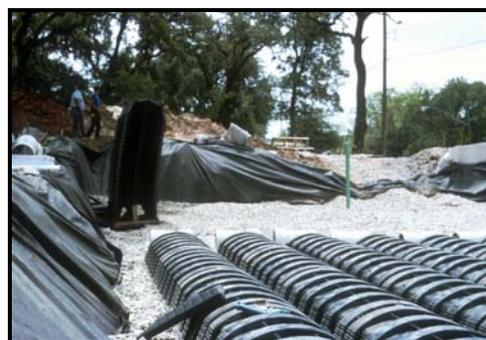
**Figure 40: Infiltration Chambers**
